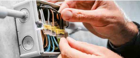
Simple and safe. The new Abox SL and SLK models simplify wiring with Wago spring terminals and thus enable vibration- and shock-proof, maintenance-free connections. Maintenance and troubleshooting are facilitated by easily accessible test openings on the terminals. The Abox SLK also has fixed-position terminal holder for more comfort during wiring and maintenance.
