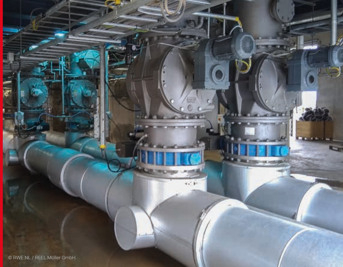
Silo discharge and conveying pipe system
