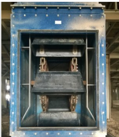
Cast polyamide buckets in the potash industry
