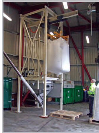
3. Traversing bag into position
