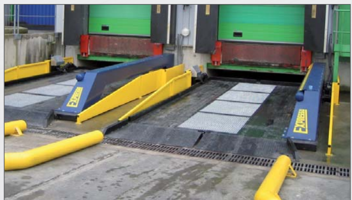
Levelling and secure immobilization
