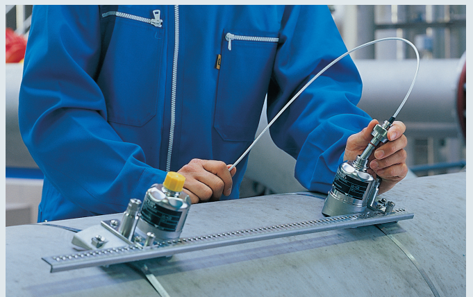
Verification of installed flowmeters
