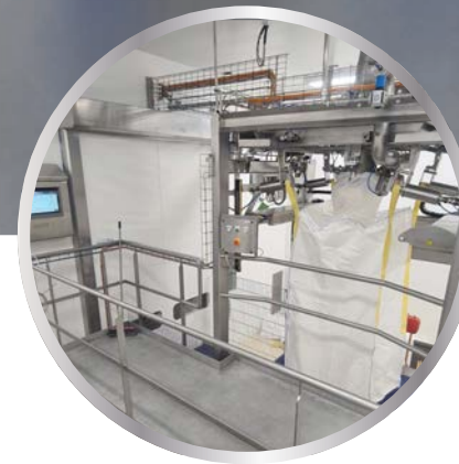
The only manual task is to connect a new big bag on to the first two hooks, the rest is automated.
