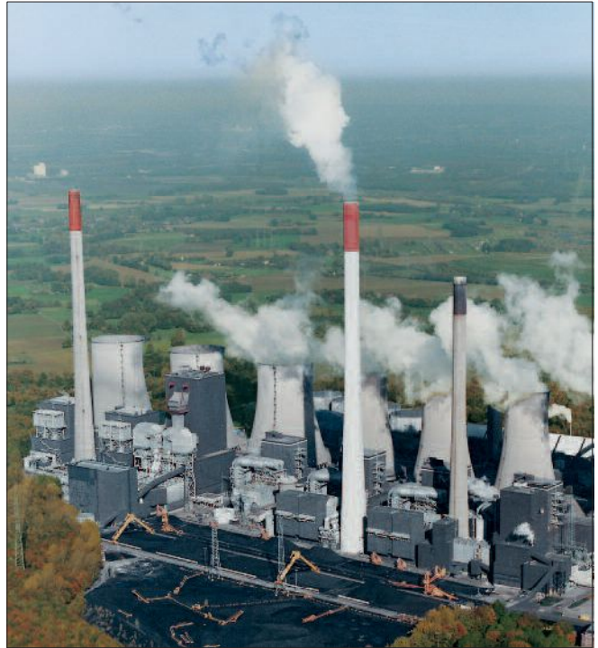
Power plant (EON)
