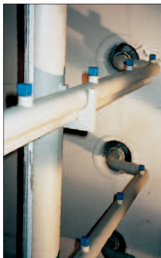
Detail nozzle spray system
