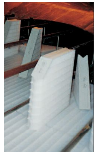
LTV 271 during installation
