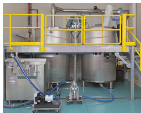
Slurry from the batching tank (R) is pumped to the feed tank (L) where it is metered into the spray dryer.
