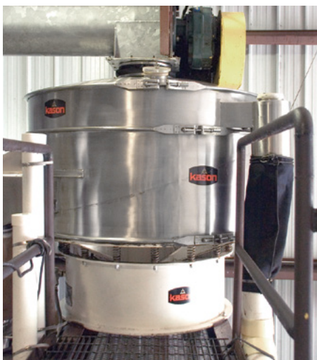
Overhead horizontal augers move sugar into the two VIBROSCREEN screeners in the facility. Each screener separates sugar lumps from grains by vibrating a single spring-mounted screening deck located in the upper part of the unit. The vibration is produced by rotation of an unbalanced-weight gyratory motor located below the screening chamber.
