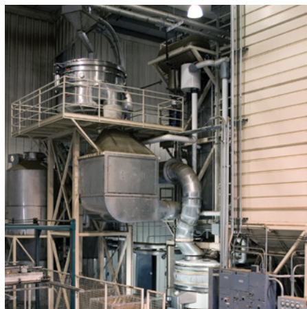
Almonds are conveyed from a holding tank (right) to a pasteurization tower (left of holding tank) from which they proceed to a fluid bed dryer (bottom) and then to a fluid bed cooler (top). Beneath the cooler is an equilibration tank where almonds achieve uniform temperature.
