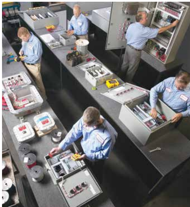
Panel assembly area of Controls Department.
