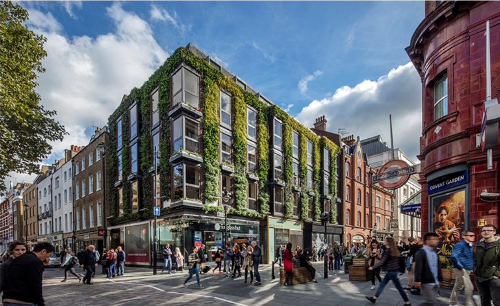
Regal House, Covent Garden, London
