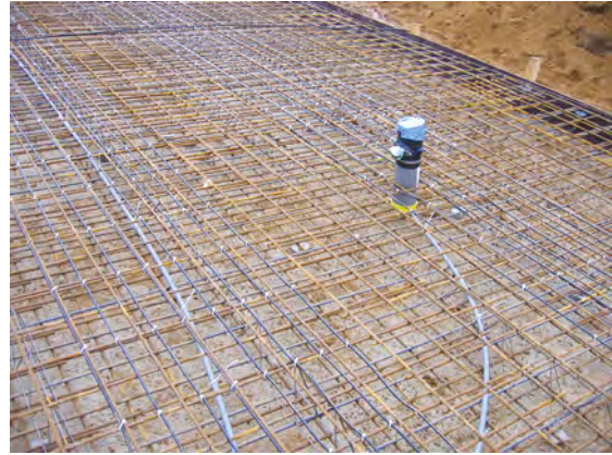
Placing the sensors
