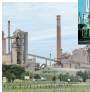
Cement and lime industry
