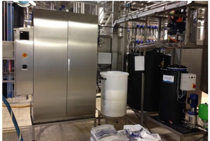
Figure 5; Dulcolyte system inside the production environment including (from left to right) generator, salt storage, HOCL storage tank, dosing pumps and water break unit.
