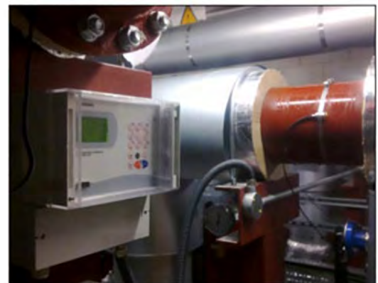
UFM-70 FS for Heat Quantity Measurement application using PT100 sensors
