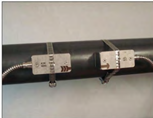
Transducers mounted using strap and clamps
