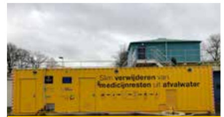
Winterswijk, Municipal Water Treatment Plant in the Netherlands (Water Authority Rijn en IJssel)
