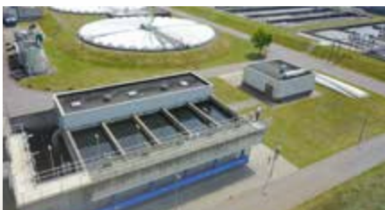
Horstermeer, Municipal Water Treatment Plant in the Netherlands (Water Authority Amstel, Gooi en Vecht)
