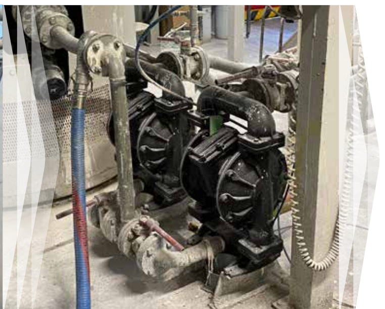
High fluid viscosity reduces pump delivery.
