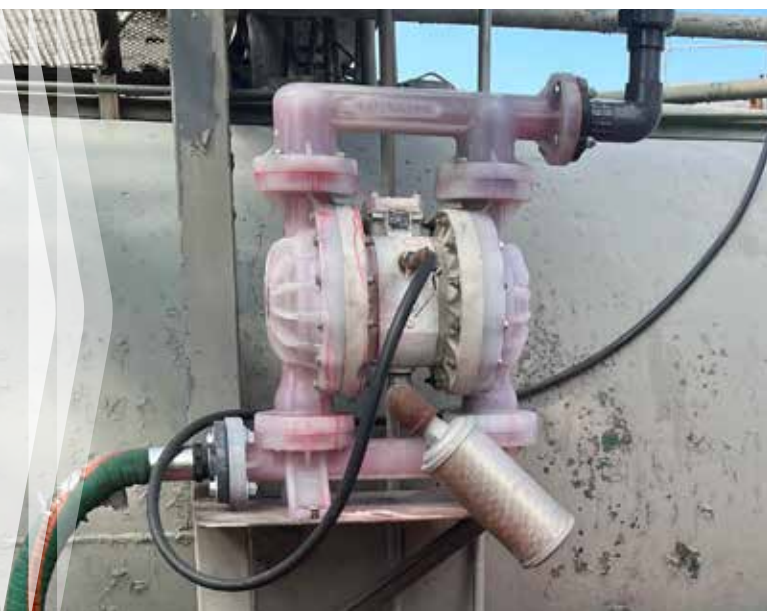
High suction lift reduces pump delivery.
