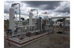
Carbis Loadtec is a leading manufacturer of Vapour Recovery Units or (VRU). VRUs are used in recovering vapours from gasoline, natural gas or other biofuels.
