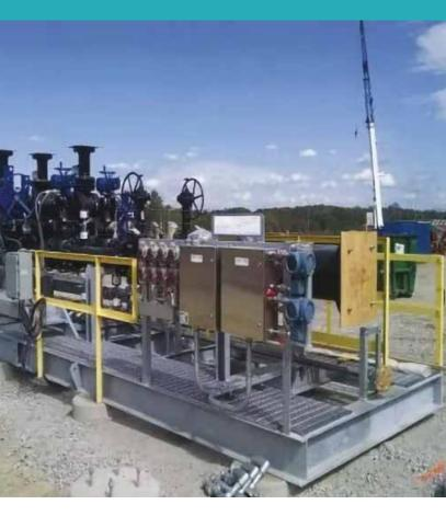
Skid frames can include spill pans, slip resistant grating walk surface with some requiring platforms with handrail and stairs on the perimeter of the skid for safe access when skids are located above grade that is not level. All meter skids are fully tested prior to shipment ensuring the skid arrives on site ready to plug/play, speeding up the installation time and allowing you to start measuring products quickly.
