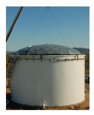
The HMT Aluminum Dome can be installed in-service.
