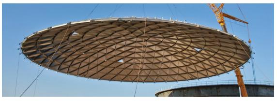
The HMT Aluminum Dome is a clear-span, lightweight, corrosion-resistant structure that sets the standard for performance in aluminum domes. The design complies with the latest edition of API 650 Annex G and the Aluminum Design Manual.
