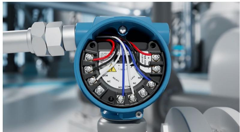
*Each relay switch consists of three terminals: Common Terminal (COM), Normally Closed Terminal (NC), and Normally Open Terminal (NO). The switch is always connected at COM and either NC or NO.*
