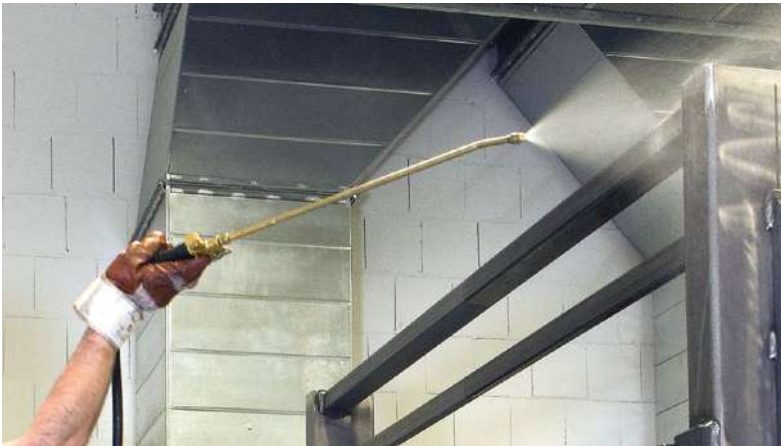
Cleaning with the FTs prior to varnishing
